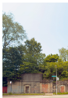
Site 3. Lake Park Node. Bronzeville Trail at S Lake Park Ave.
